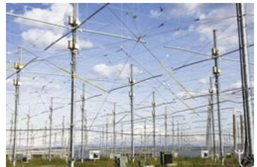
The High-frequency Active Auroral Research Program facility Gakona, Alaska. The 33-acre ionospheric research instrument helps researchers study the ionosphere. [JR Ancheta, photo]
