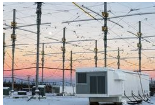
A section of the extensive HAARP antenna array and one of the transmitter shelters. [Photo courtesy of Jeff Dumps, KL4IU]
