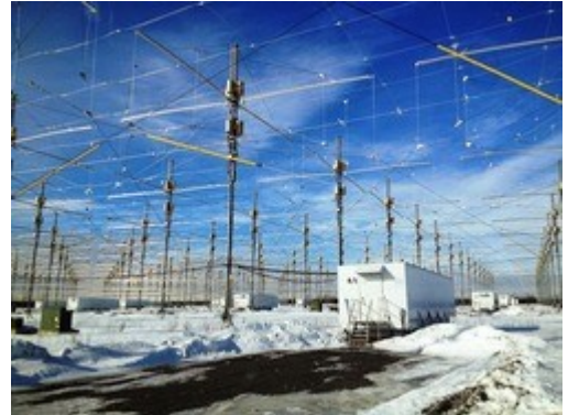
A closer look at a portion of the HAARP antenna array. The white buildings house transmitters.
