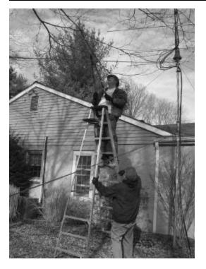
This last photo shows me, KB1JEY, trimming some interfering branches and the erected mast and antenna, guyed with my ample collection of Harbor Freight blue poly rope and Home Depot rebar stakes.
