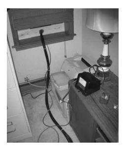
This shows my improvised window feed-thru for the coax and rotor cable. Air conditioning foam does wonders for sealing out the cold.
